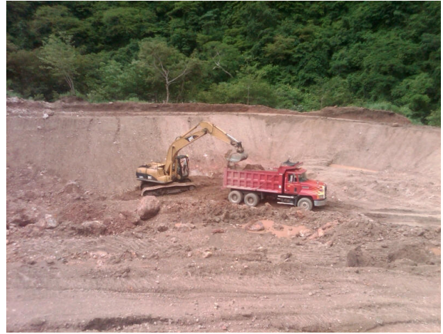
Excavation work May 2011
