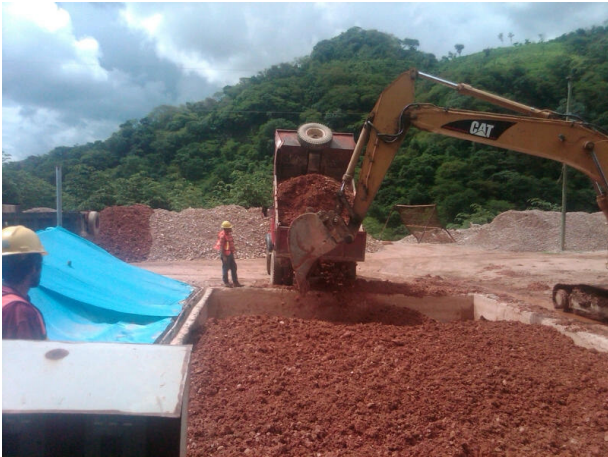
Small leach pad topped up with ore
