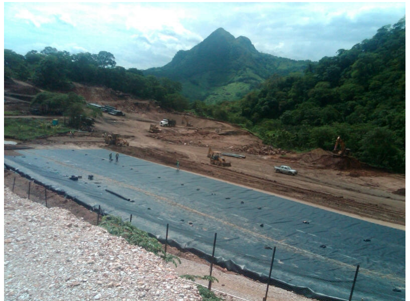
Leach pad construction nears completion
